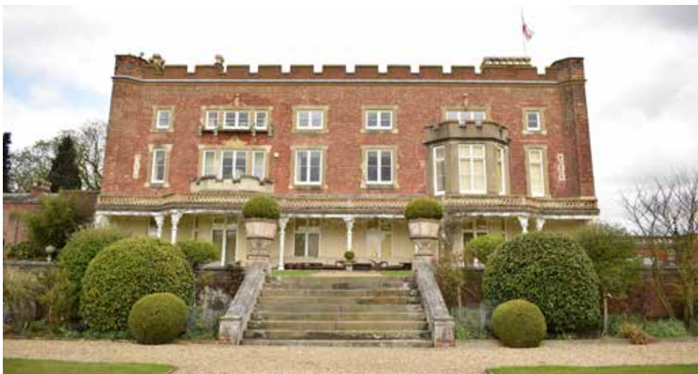
A1.5 – The principal south elevation of Hunsdon House with a first floor oriel window to the right and wide tripartite window ranges to the left. On the ground floor is a verandah. These features all help to illustrate the relationship of the house to its garden setting with 'picture' windows designed to afford a view over the garden and lakes and the countryside beyond. The land beyond the lakes and the Wellingtonia was once part of the park to Hunsdon House and would have been designed to form part of the view. The development proposed on this land will be very evident – the built forms and associated infrastructure (lighting for example) will be visible the nature of the urban form and function will be apparent by the noise generated and the knowledge that development sits so close and on land that previously formed part of the park will alter the perception of the place as a Country Estate and the hub of three medieval deer parks.
