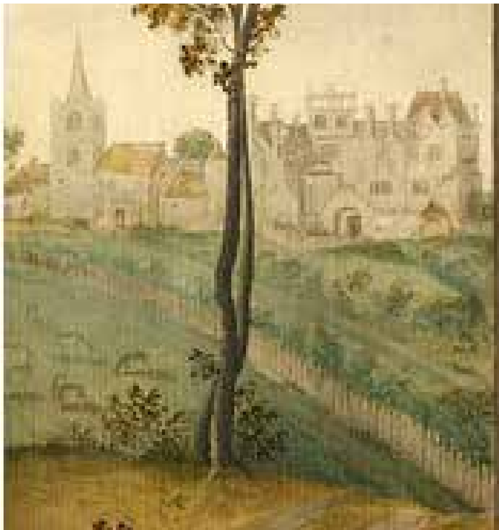
A2.1 - Hunsdon Royal Palace, grounds, Deer Park, and St Dunstan's Church 1546 from the south west.
