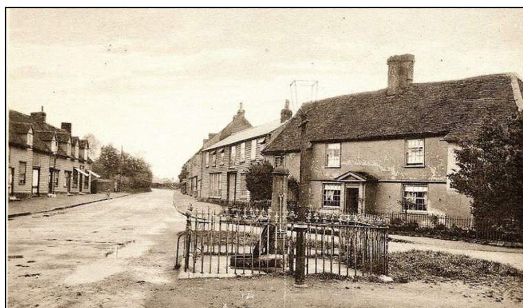
Figure 6: Hooks (later the Pump House)
